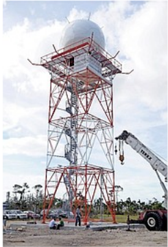
The newly-installed WRM 200 doppler radar at the weather station at LPIA. Photo: Shawn Hanna/Tribune Staff
