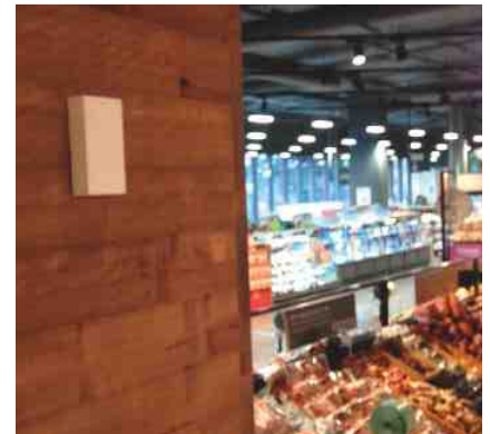
Vaisala HMW90 series transmitter on the wall.
